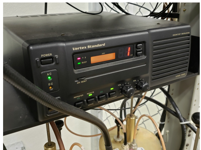
This is 1 of 2 Vertex VXR 7000 repeaters we own on Channel 1 memory (set to 82/22)
