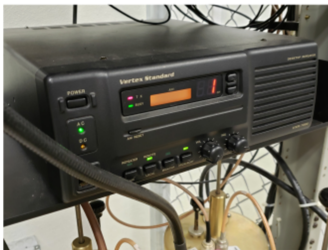
This is 1 of 2 Vertex VXR 7000 repeaters we own on Channel 1 memory (set to 82/22)
