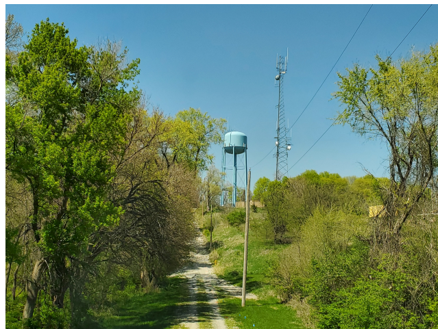
This is the Memorial Park / Gleason St site, a 200 ft tower beside original .22 water tower
