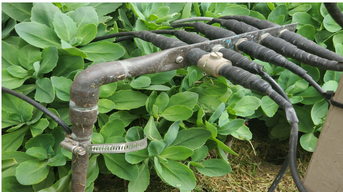
Figure 1: Coax ground at KD0YTI's Shack
